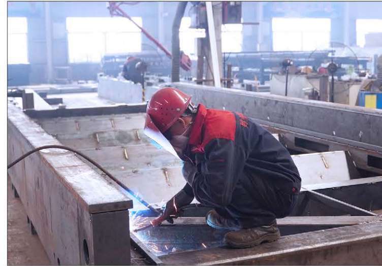
坡口焊接 | Groove welding
